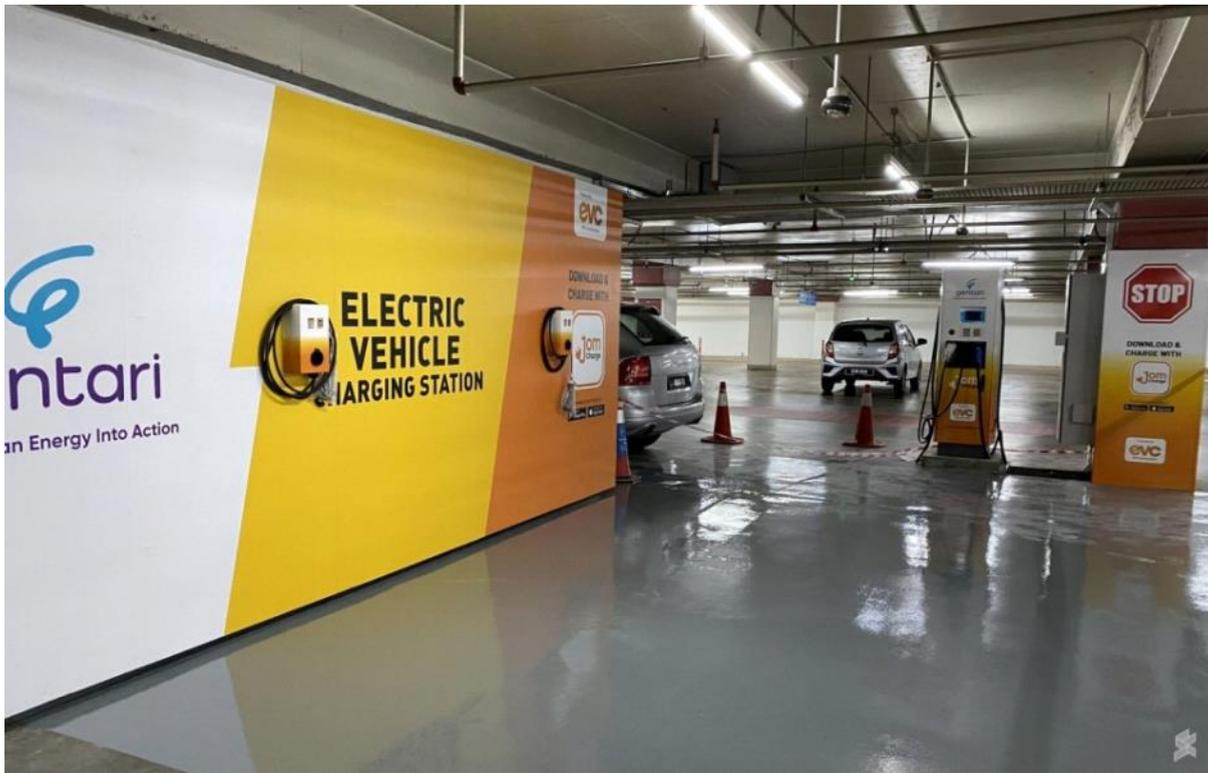
The new EV charging station by [Gentari](#) and [JomCharge](#) is located near the Southcourt travelator at (around Pillar A43) Level P2, Mid Valley Megamall carpark. For fast charging, there's an ABB Terra 54 DC charger which can push up to 50kW. This unit has a total of three nozzles which include Type-2 AC as well as CCS2 and CHAdeMO DC connectors. This station also has two AC charge points which is great if you plan to leave your EV for a couple of hours.
