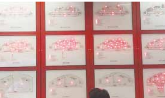
Fire alarm system upgrade with LED indication
