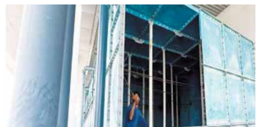
Replacement of water tank tie rod & water tank cleaning at Centrepoint North and South
