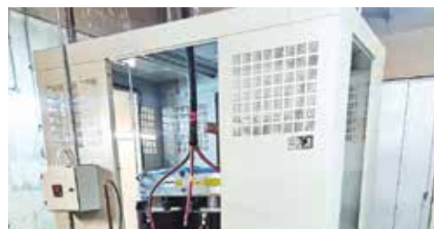
Transformer replacement at Mid Valley Megamall
