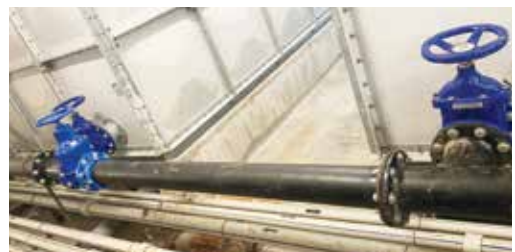
Bypass pipe between the flushing tank and the drinking tank to cater for emergency such as water disruption at Southpoint Offices & Retail
