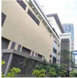
Repair and repainting of East Entrance Façade
