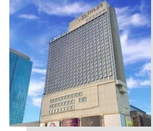
St Giles Hotel, Southkey Johor Bahru (575 rooms)
