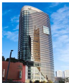
The Gardens South Tower Value: RM398 mil
